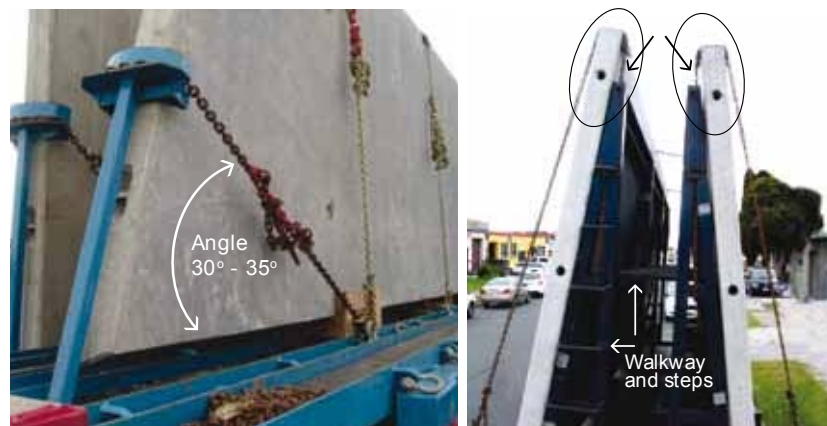
Figure 2, Safety chains example: 4 chains with 2 front chains independently holding each panel.
