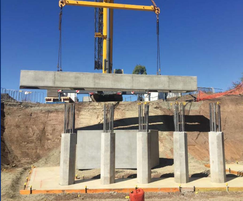
Stresscrete prides itself in its commitment to delivering quality products on time and this bridge was no exception. Prestressed piles and deck units, lower abutment blocks and abutments, lower wing wall blocks and wing walls were manufactured for the bridge. Mr Zinn says the piles and deck units were cast in the factory's in-line stressing bed, while all remaining precast was manufactured using traditional methods utilising timber formwork.
