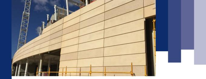
According to Mr Ferraro, the stadium seating project has been challenging in terms of both its design and tight timelines. At the peak of production 25 units were being manufactured every day. "There were 900 different unit types so repeatability of the product was minimal. They're all configured slightly differently, some with variations of as little as five or 10 millimetres. That is to ensure sight lines, so everyone, no matter where they are sitting, can have a great view".
