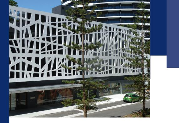
A further degree of difficulty was that the bulk of the panels had subtly different shapes, due to the shaft and the head size changing on each level, requiring use of more than 20 moulds and calling for a mould change in one out of every three panels cast. In fact, the project called for a staggering 518 different panel shapes.
