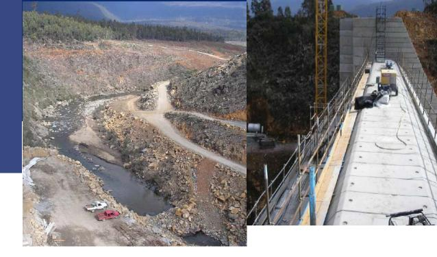
Panels were generally poured before 2.00 pm, so they could be lifted before 7.30 am the following day. Prior to lifting, the moulds were released and eye bolts placed in ferrule holes.
