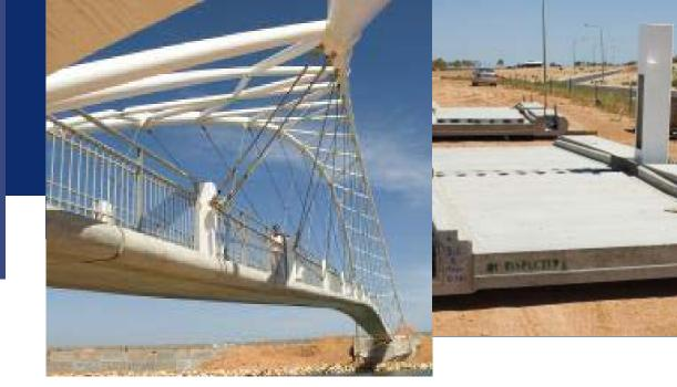
Meanwhile, precast manufacturer Delta Corporation was completing the precast decking units that would provide essential structural stability against cyclonic wind uplift as well as forming the 1.8 metre wide footway. Precast deck units, apart from aesthetic considerations, were selected for the steel arch structure to provide sufficient mass to stabilise the structure against wind uplift prior to the grouting-in of stressing cables that perform this task in the completed structure.
