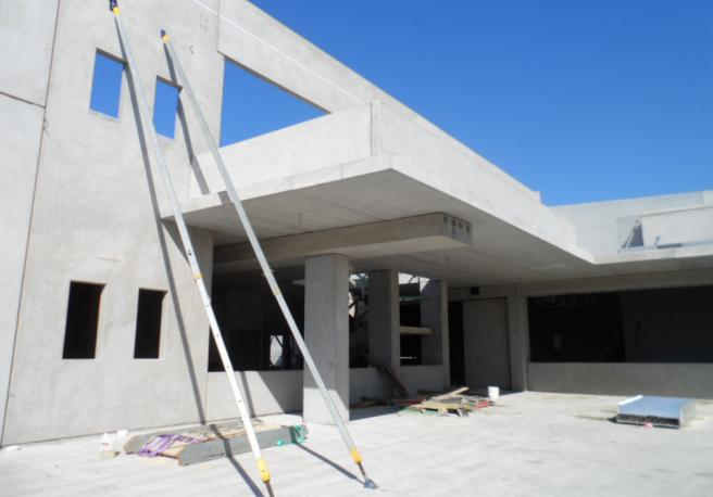
"Using precast prestressed beams and flooring gave greater spans, enabling a reduced number of columns," he details.
