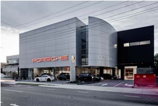
Porsche showroom - Hollowcore Core Concrete, VIC
