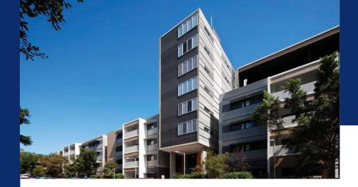
"Sandwich wall panels which were typically 260mm thick were supplied, although 280mm and 310mm panels were also supplied," explains Chris Parsons, Manager for Hanson Precast, which was contracted to make and supply the precast components.
