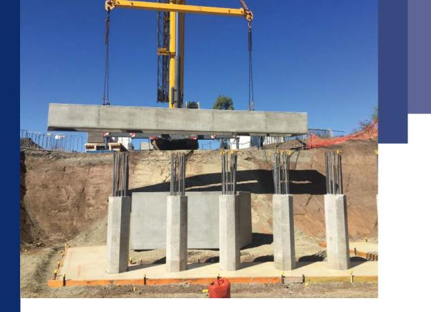
Stresscrete prides itself in its commitment to delivering quality products on time and this bridge was no exception. Prestressed piles and deck units, lower abutment blocks and abutments, lower wing wall blocks and wing walls were manufactured for the bridge. Mr Zinn says the piles and deck units were cast in the factory's inline stressing bed, while all remaining precast was manufactured using traditional methods utilising timber formwork.
