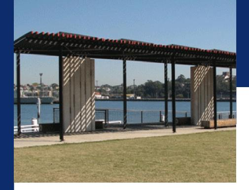
Hanson Precast was selected to provide the playground's barbecue benches, seating areas, flat steps, paving areas, spacers and columns. These were finished in a Class 2 off-form concrete, using off-white cement, as were other new elements. These included 'boomerang' concrete walls that sculpt the grove to ensure they are integrated with the original elements of the restored area.
