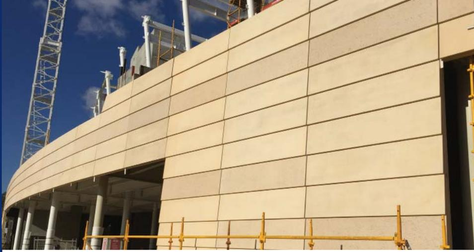
Although specified as a Class 2 finish, the finishes to the panels are Class 1 off-form, in earthy tones with a saw tooth profile. Special custom moulds were fabricated specifically for the project. Different depths of sand blasting to selected segments give the panels unique and contrasting architectural finishes with some smooth and others with exposed stone.
