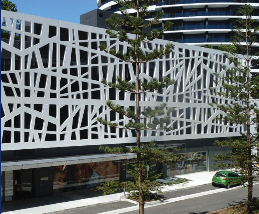
A further degree of difficulty was that the bulk of the panels had subtly different shapes, due to the shaft and the head size changing on each level, requiring use of more than 20 moulds and calling for a mould change in one out of every three panels cast. In fact, the project called for a staggering 518 different panel shapes.
