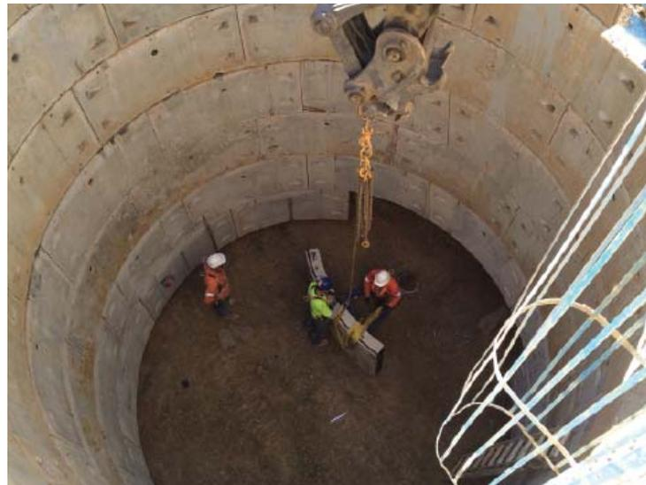
Precast segmental shafts for the sewer were also manufactured at the company's factory in Echuca in country Victoria. The shafts were supplied to Rob Carr, installers of underground pipes and services and sub-contractors to Lend Lease.
