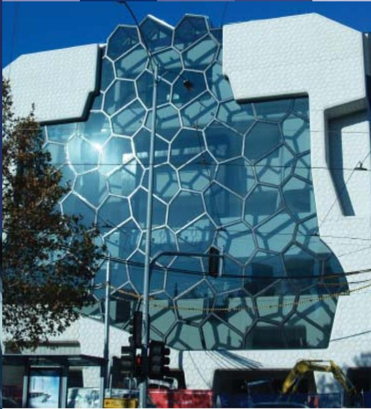
Lightweight – at a slender 25mm its panels can be cast thinner than those of conventional precast – and strong, it was both a cost effective and environmentally sustainable choice. It also has excellent acoustic properties, blocking both street noise and enhancing the quality of the performance space within.
