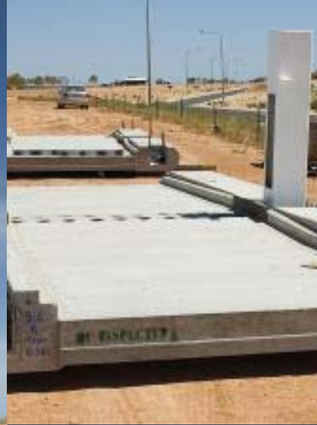
Meanwhile, precast manufacturer Delta Corporation was completing the precast decking units that would provide essential structural stability against cyclonic wind uplift as well as forming the 1.8 metre wide footway. Precast deck units, apart from aesthetic considerations, were selected for the steel arch structure to provide sufficient mass to stabilise the structure against wind uplift prior to the grouting-in of stressing cables that perform this task in the completed structure.
