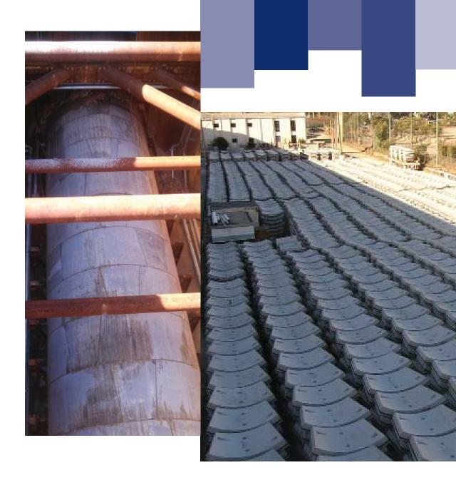
Director Ian Coulter says precast concrete was chosen to ensure reliable delivery, easy segment installation and a high quality finish. "We had to specially manufacture a huge 22,000 concrete segments for the tunnelling," he said.
