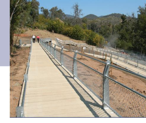
Following community feedback, a discovery trail was designed and installed to allow access by the public to get a better and safer viewing location of the construction process at the new dam wall. The boardwalk system was used to connect the elevated viewing platform to the river trail below via gently graded accessible sections, with stepped 'short cuts'.
