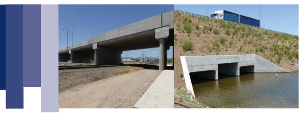
This particular stretch of highway featured a bridge over Sturt Creek, which required 34 prestressed bridge decks. The new 27 metre two lane bridge was constructed next to the existing bridge, which was then demolished to then construct a second bridge, providing two lanes for both directions. The two new bridges are higher than the previous one, reducing the risk of flooding and flood damage to the bridge.
