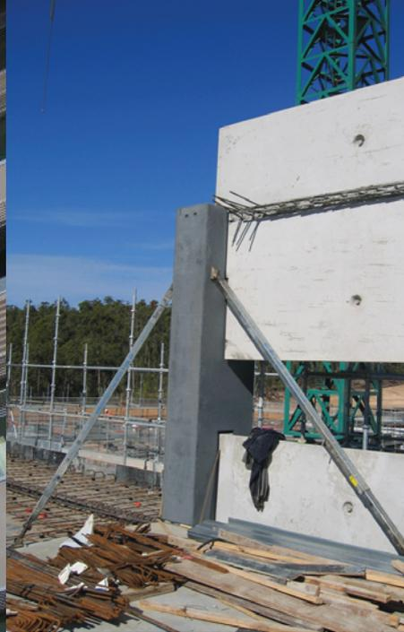
Of equal benefit to the builder as the reduced time, the site workforce for the building structure was drastically reduced and consisted primarily of a precast erection crew, form worker to place the metal deck floor system and a concreting crew to pour the floors.
